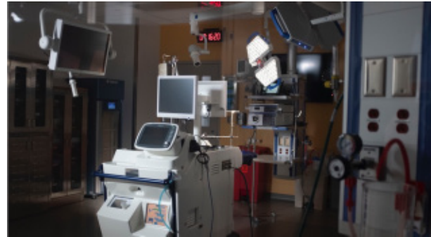
FIRST OF ITS KIND FACILITIES
